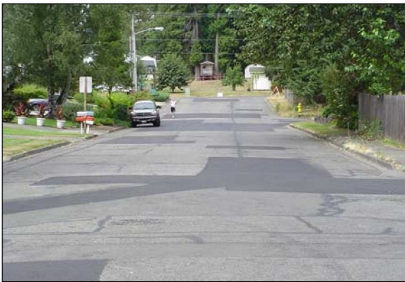
Save Our Streets - Patching Treatment
