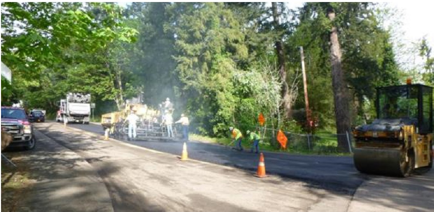
Figure 2: S 288 th Street grind and overlay
