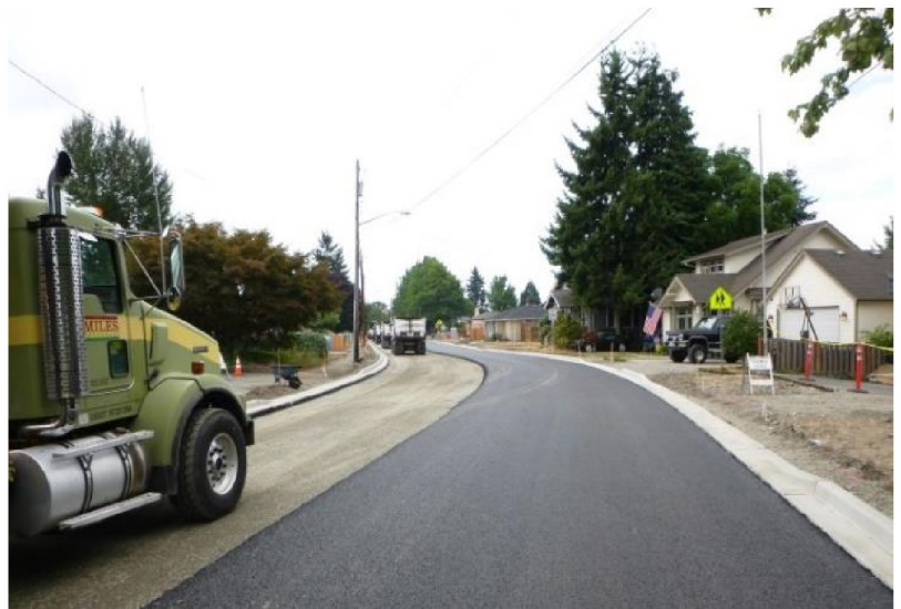
Figure 3: Street Reconstruction of D St SE between Auburn Way South and 12th St SE
