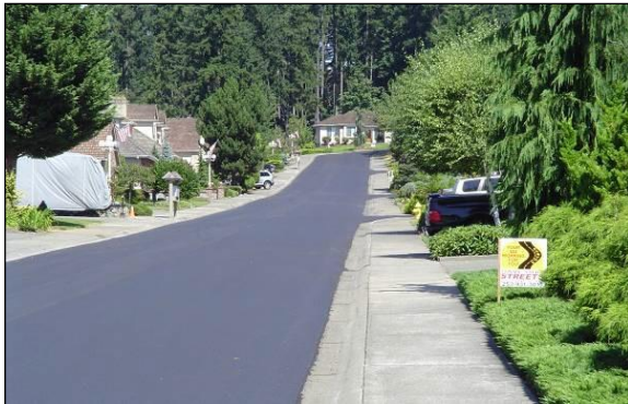
— Save our Streets – Patching Treatment Save our Streets- Overlay
