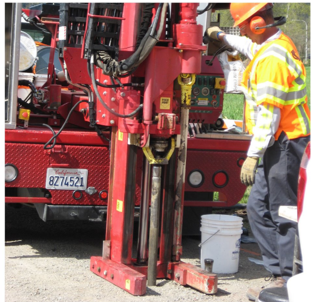
Drilling for groundwater samples in northeast Algona.
