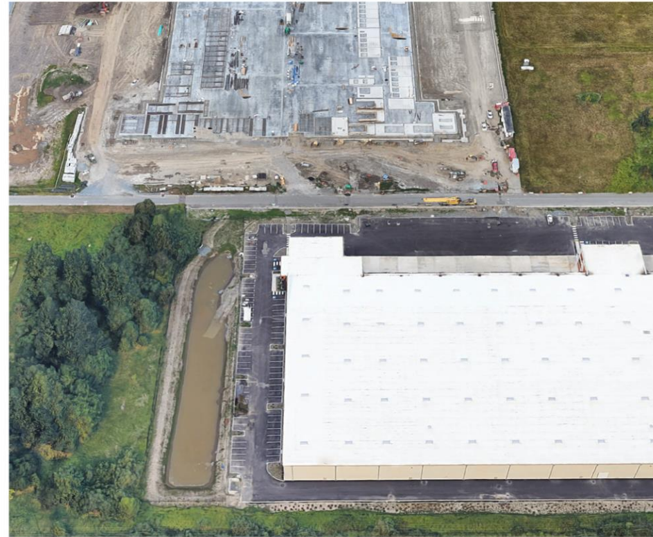
New Warehouse Development, with fill brought in and addition of flood storage facilities
