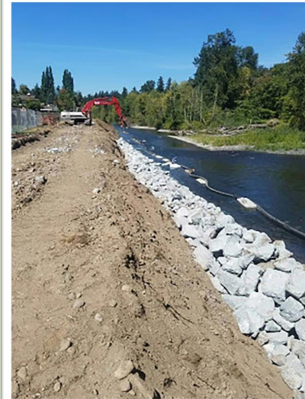
Flood protection projects, such as repairs to existing levees
