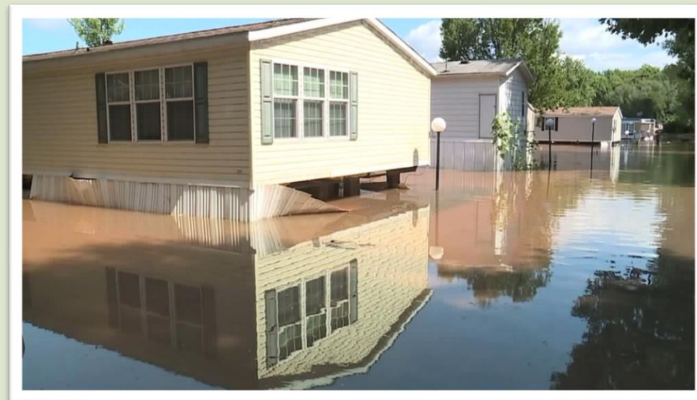
Example of Manufactured home built above flood elevation
