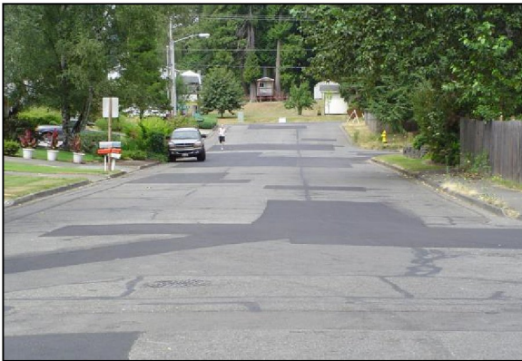
Save Our Streets - Patching Treatment
