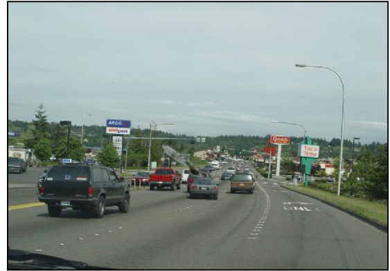
Principal Arterial: 15th Street NW
