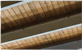
ORIGINAL WOOD CEILING
