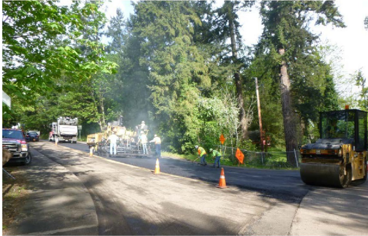
Figure 1: XXX Street Grind & Overlay
