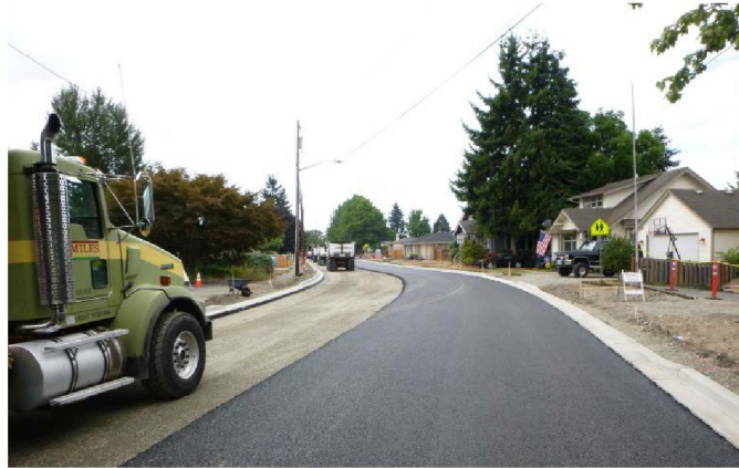
Figure 2: Grind & Overlay XXX St SE
