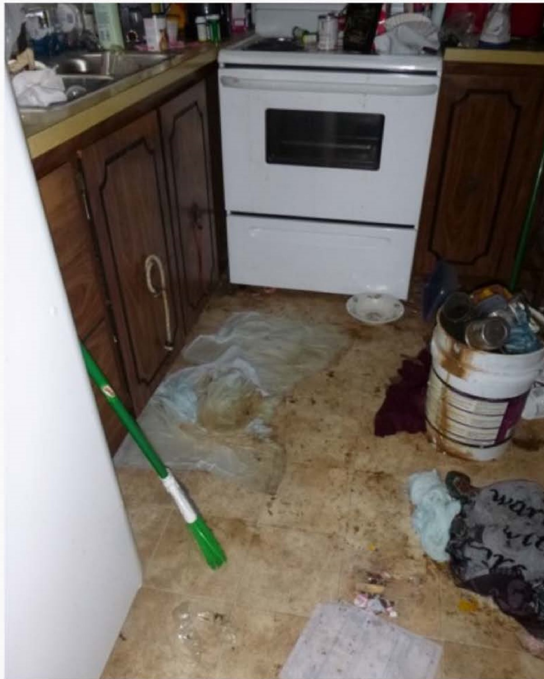
JANUARY 2016 | Leaking pipes in the kitchen
