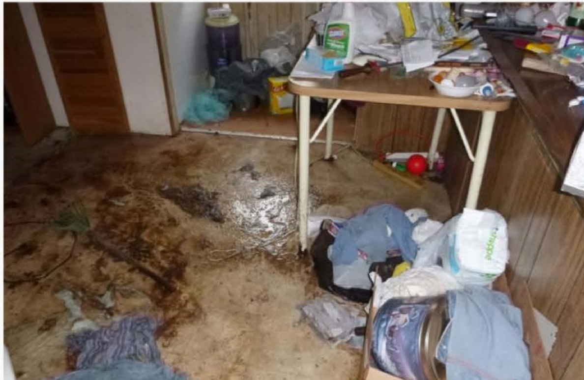
Building inspector conducts home visit and requests assistance
