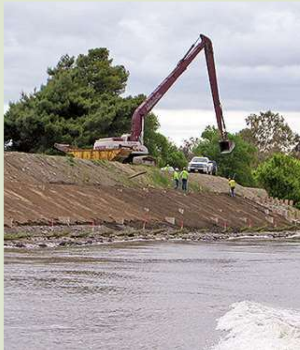
Construction of new levee system
