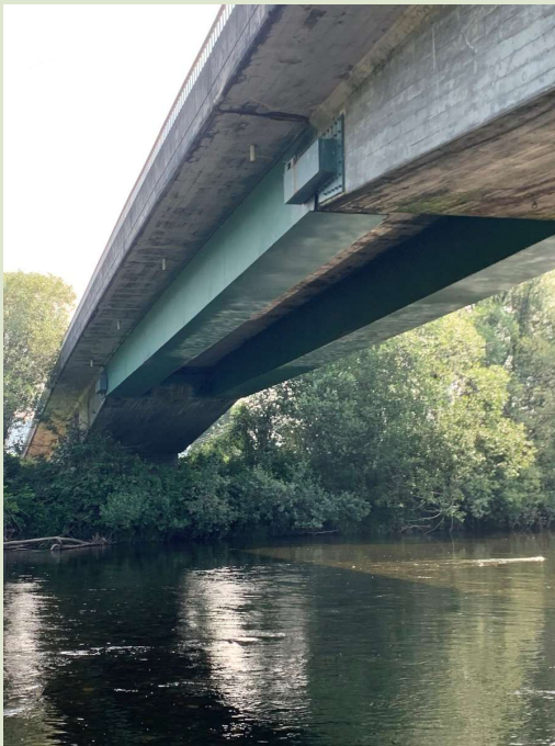
Construction of new over-water bridges
