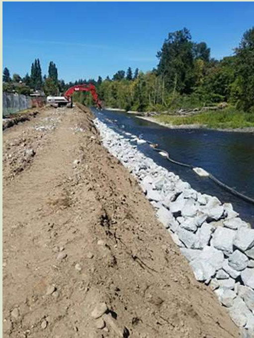
Flood protection repair or enhancement projects, such as levee repairs
