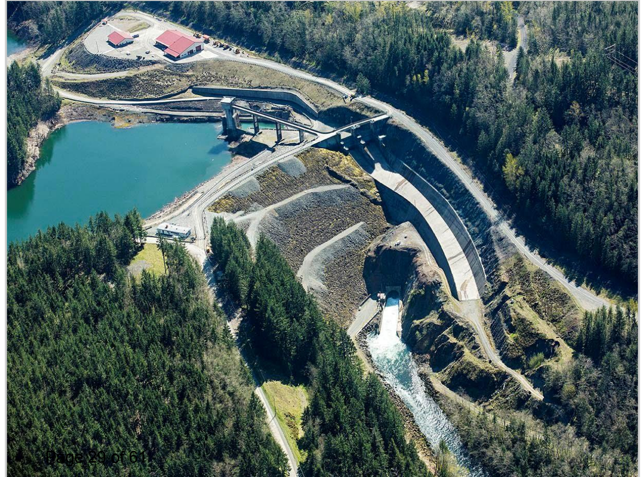
Howard Hansen Dam Fish Passage
