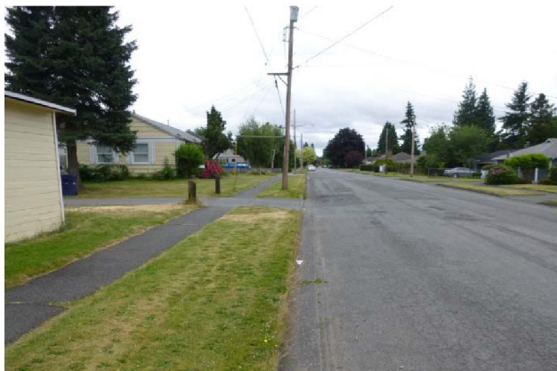
K St NE Before Rebuild
