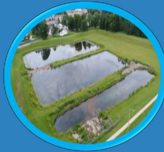
Storm water management
