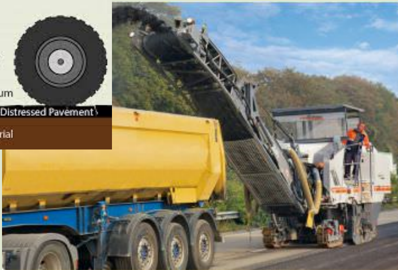
Removal of material
