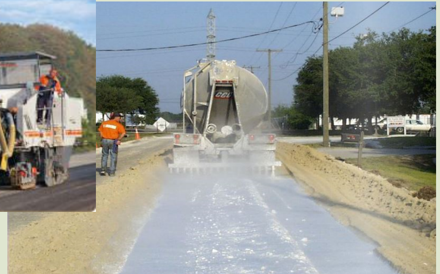
Application of stabilizing Cement
