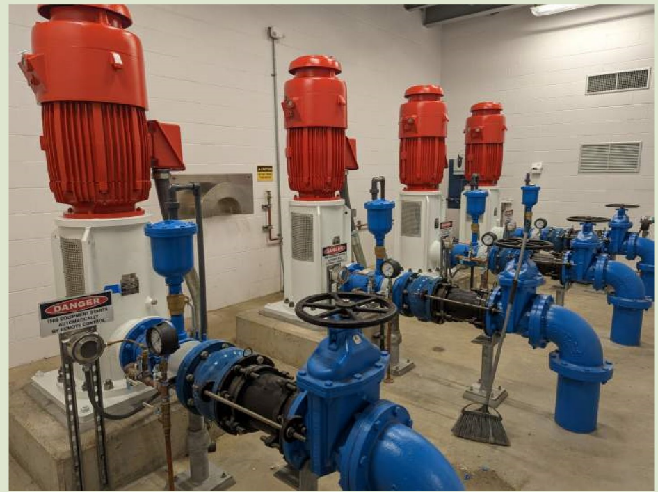
Academy Pump Station
