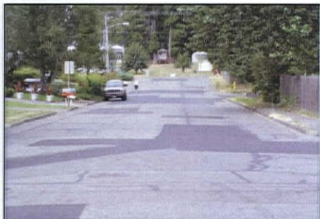
Save Our Streets - Patching Treatment
