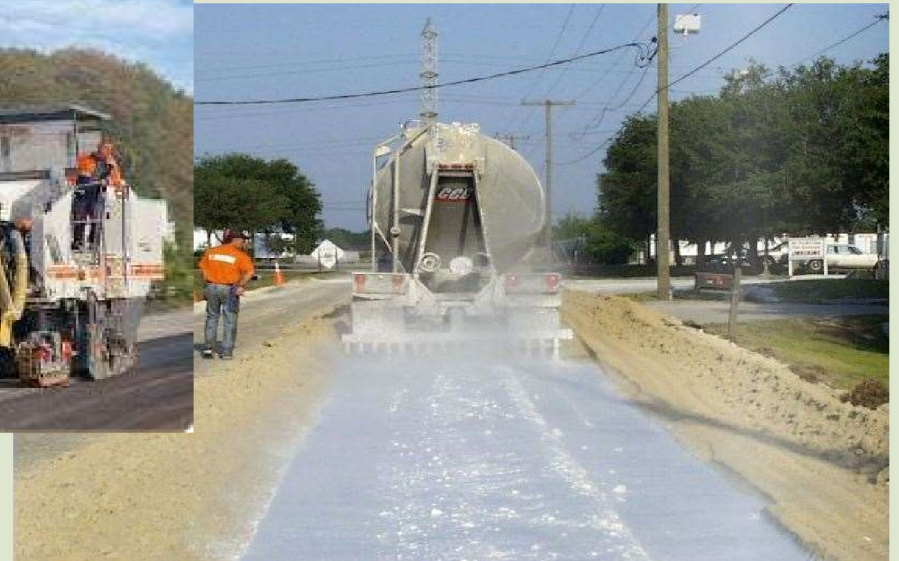
Application of stabilizing Cement
