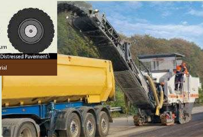
Removal of material
