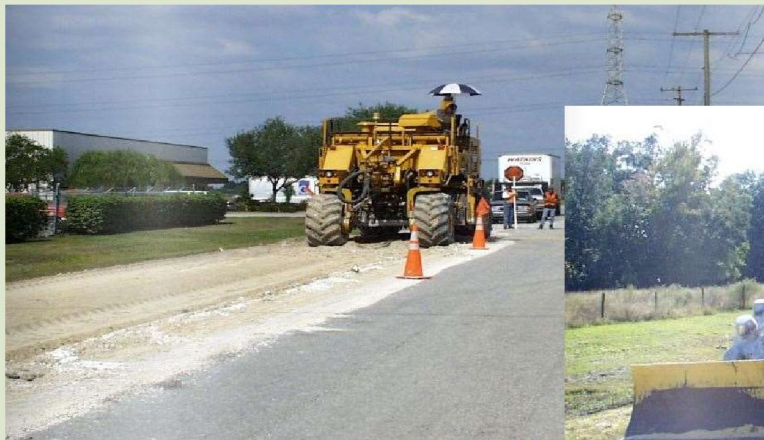
Blend in stabilizing material
