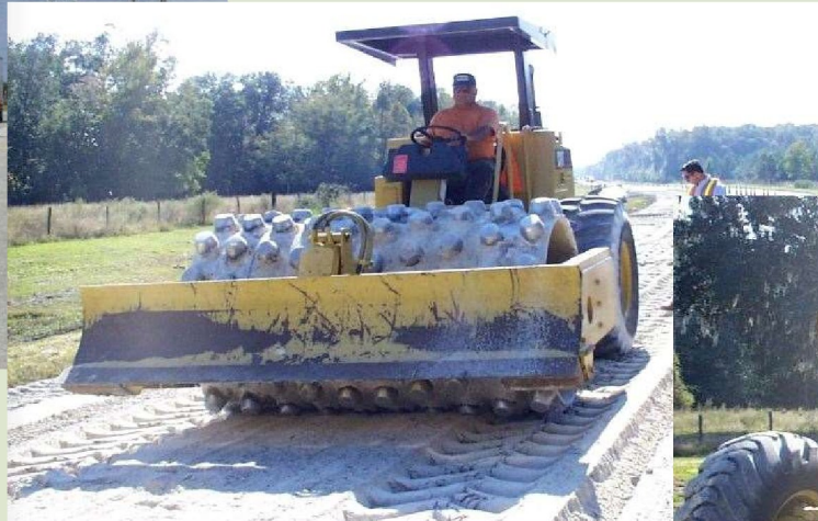
Compact the subgrade
