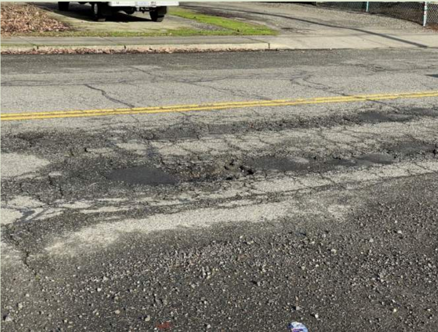
Failing Pavement
