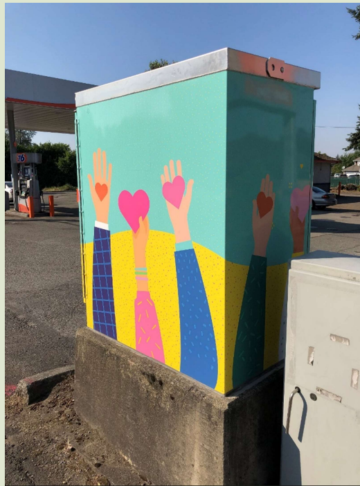
Auburn Way S / Academy Drive
