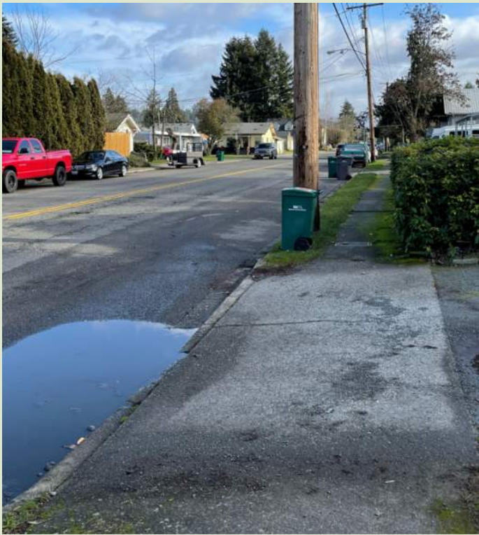
Left – Standing Water/Drainage Issues.
