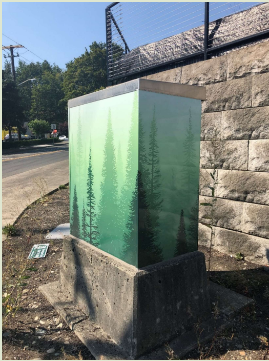
West Valley HWY / 37 th Street NW
