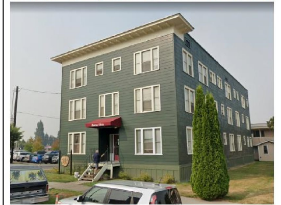
Repainted building with period paint colors, added awning, and sign with wood from removed tree
