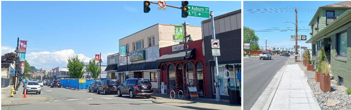
L: Vehicle traffic and construction on E Main Street. R: Five-foot sidewalks on Auburn Way N.
