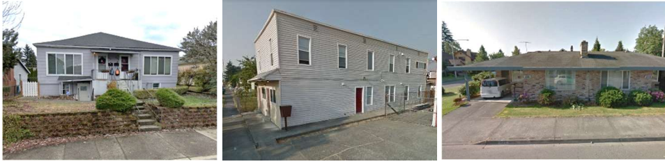
L-R: Existing nonconforming triplex, six-plex, and duplex in downtown Auburn. Source: Google Street View © Google
