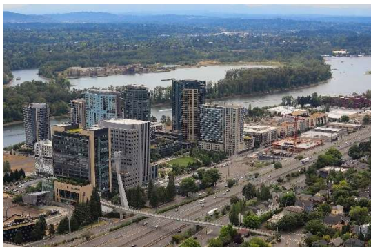
OHSU anchors redevelopment in Portland South Waterfront neighborhood.
