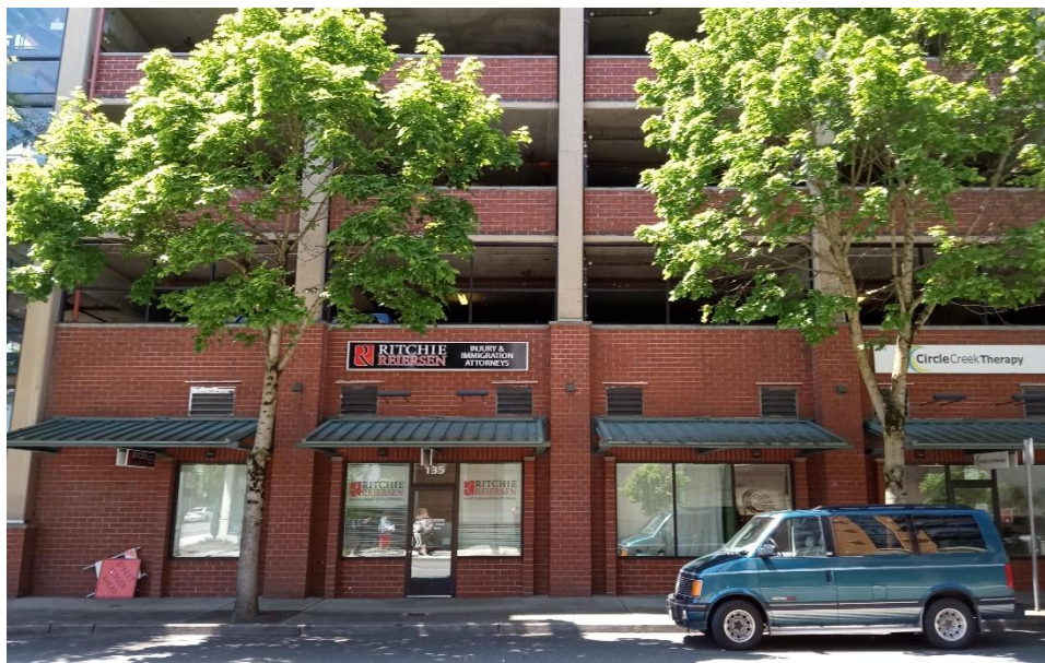
Auburn Station Park and Ride Garage
