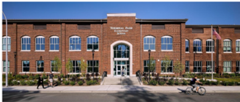
Terminal Park Elementary School – 2023
