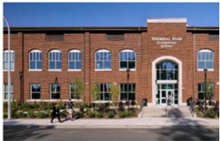
Terminal Park Elementary School – 2023
