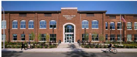
Terminal Park Elementary School – 2023
