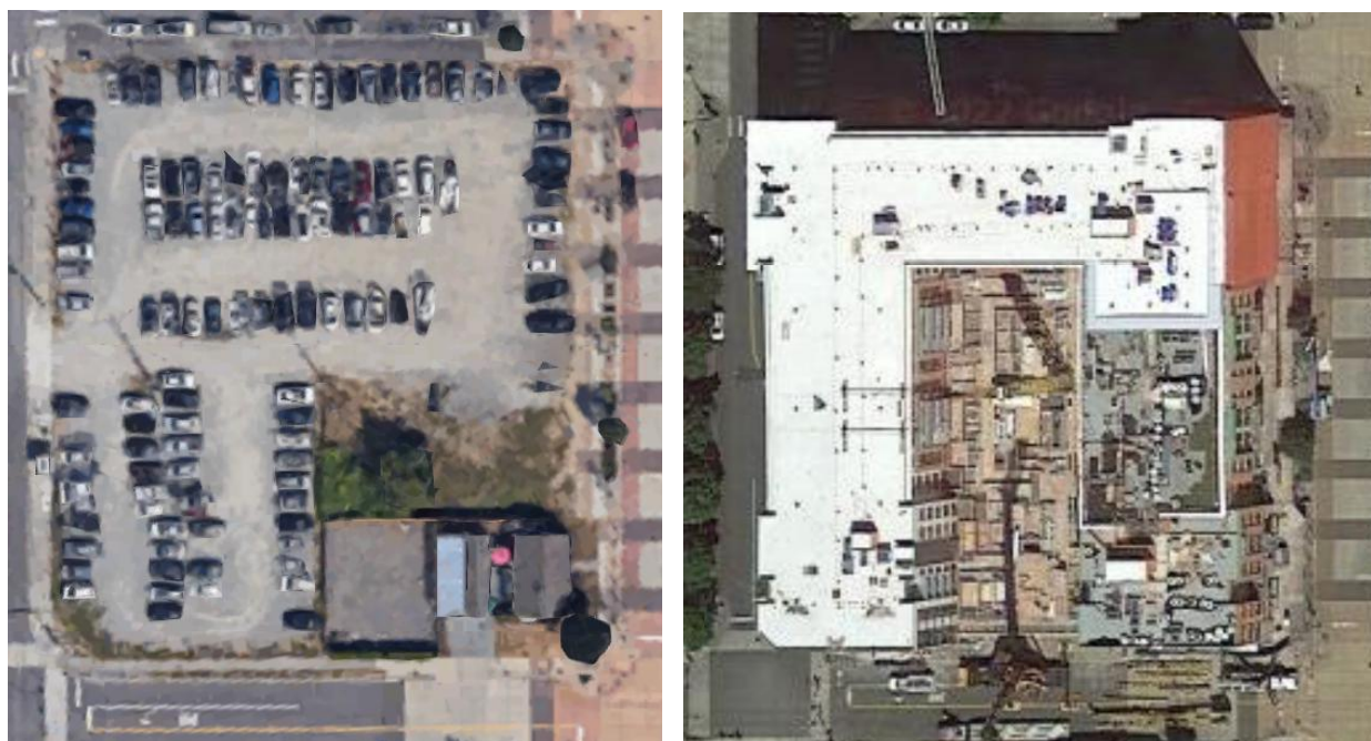
FIGURE 6-18 The Verge Apartments Before and After Development
