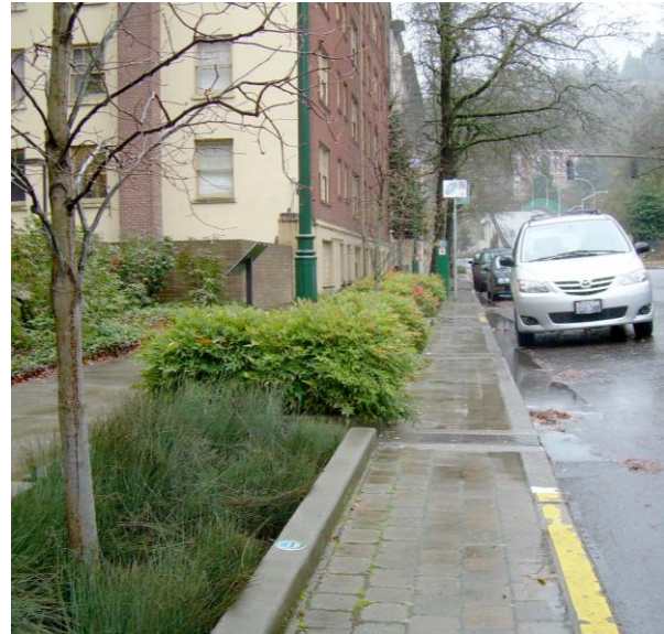
Examples of green stormwater infrastructure integrated with private development (at left) and incorporated into a streetscape (at right).
