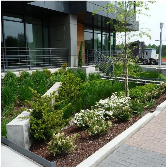
Examples of green stormwater infrastructure integrated with private development (at left) and incorporated into a streetscape (at right).
