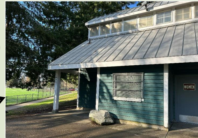
GAME FARM RESTROOM REPLACEMENT
