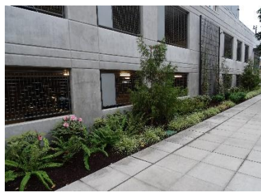
Parking garage with windows
