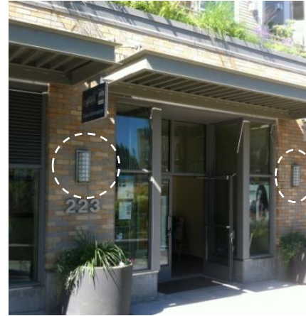
iii: Decorative light fixtures.
