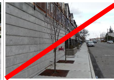
Parking garage without windows
