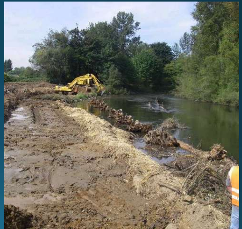
Fenster Levee Setback, Auburn
